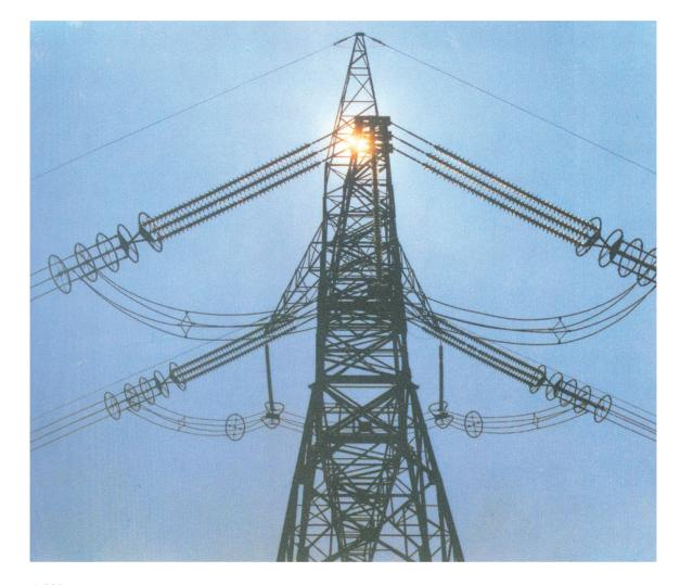
ACSR has long been the backbone of overhead transmission and distribution systems. It has altogether replaced older types of overhead conductors made of copper, which are now a days used only to meet specific demands.
