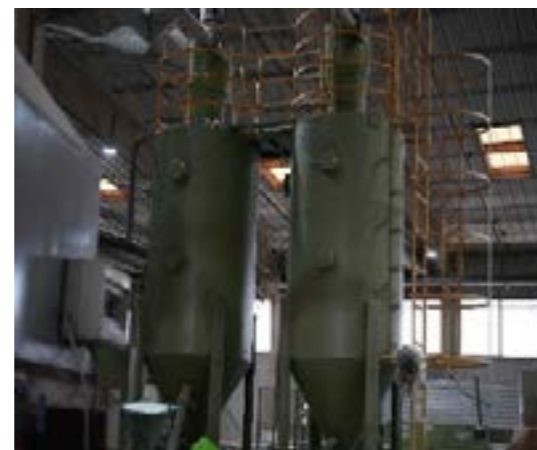
Figure 8. Water Coolers in the Factory
